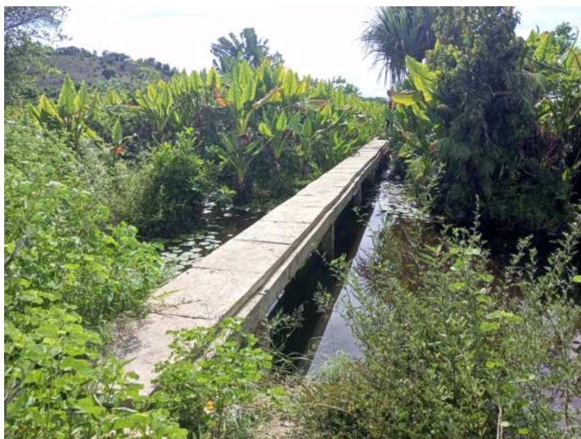
Footbridge in detached parcel Andranoanala , December 2024, © WCS Madagascar
